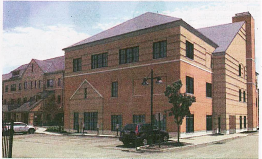
ABOVE: Artist's rendering showing the vertical expansion of the west wing of Children's Home of Pittsburgh. Photo courtesy VEBH Architects
